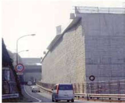
Fig.11 Completed wall with cantilever portion.
